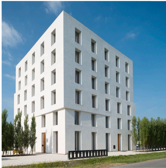
Fig. 3. View of the reference building (Source: exterior view Building 2226 Norbert Prommer).
