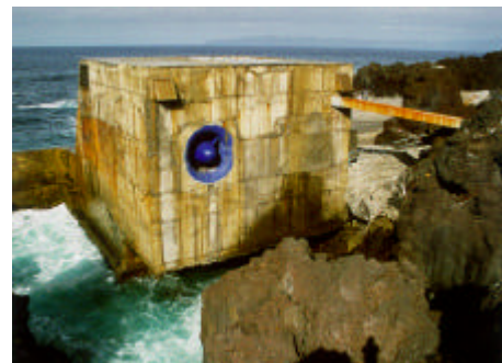
400 kW (1998), Pico Island (Azores) Fully automated, full-scale testing facility
