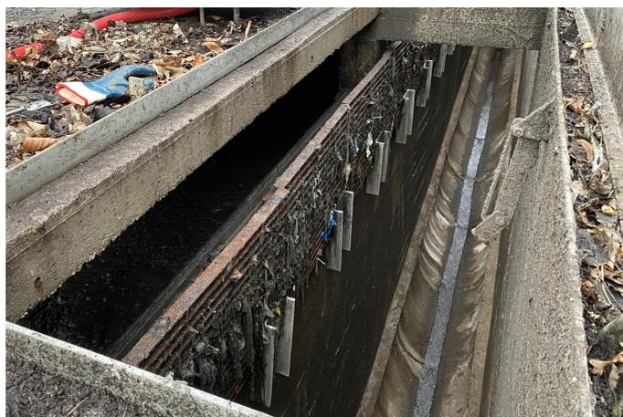
**Figure 10.13.** Photo of the screen at the CSO structure at Thulevej. The photo was taken after an attempted cleaning of the screen [Sørensen, 2022].
