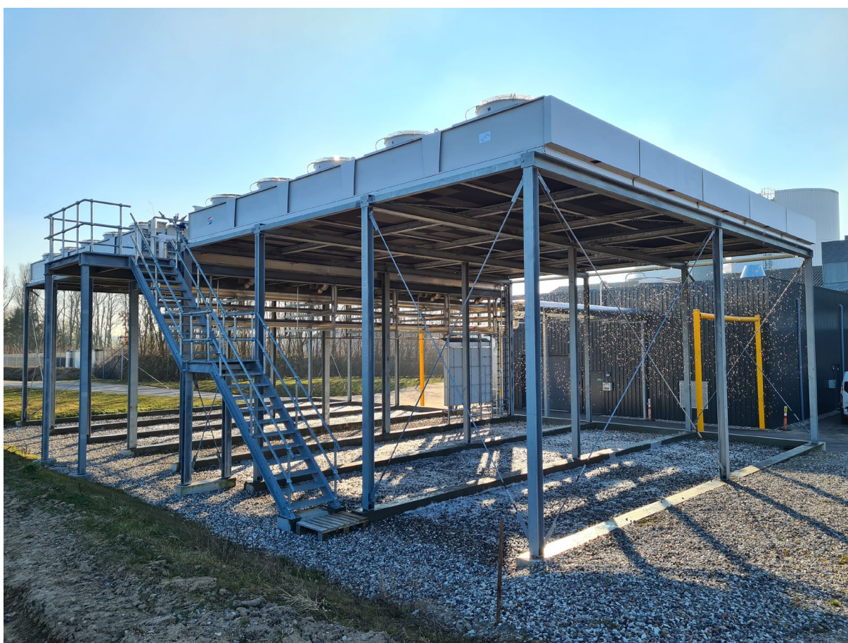
Figure 5: Flatbed air coolers of the 3 MW heat pump at Præstø Fjernvarme, Denmark; source: Daniel Trier (PlanEnergi).
