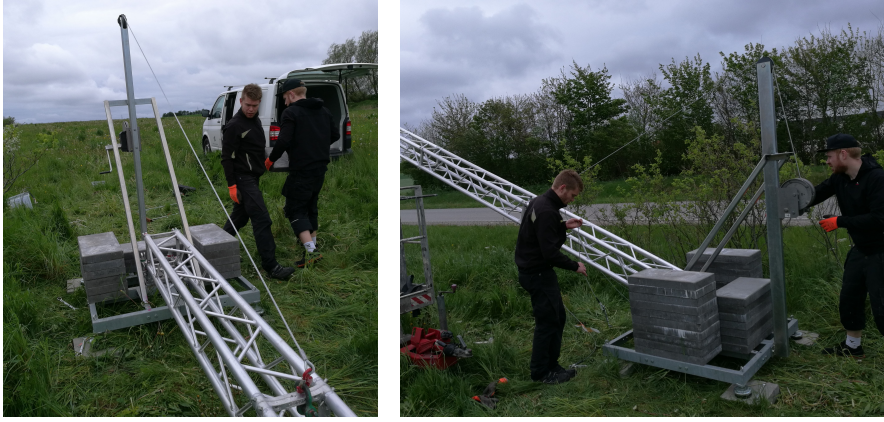
Fig. B.13: The portable pole can be raised using a swivel bracket installed in the middle of the base platform. The pole is raised using a steel wire connected to a manual winch system.
