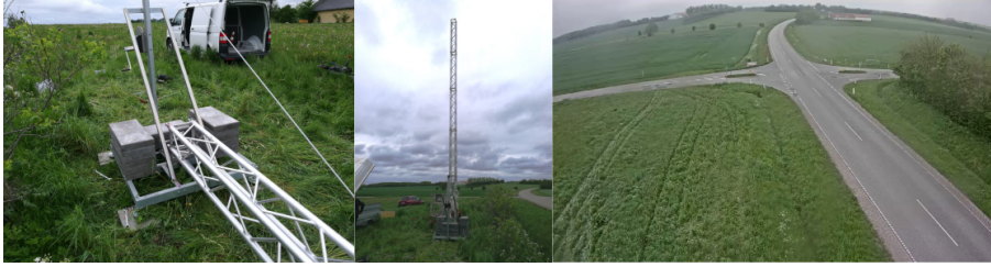
Fig. 2.11: The TRG-pole is deployed at a traffic intersection with limited existing infrastructure. Image source: [1].
