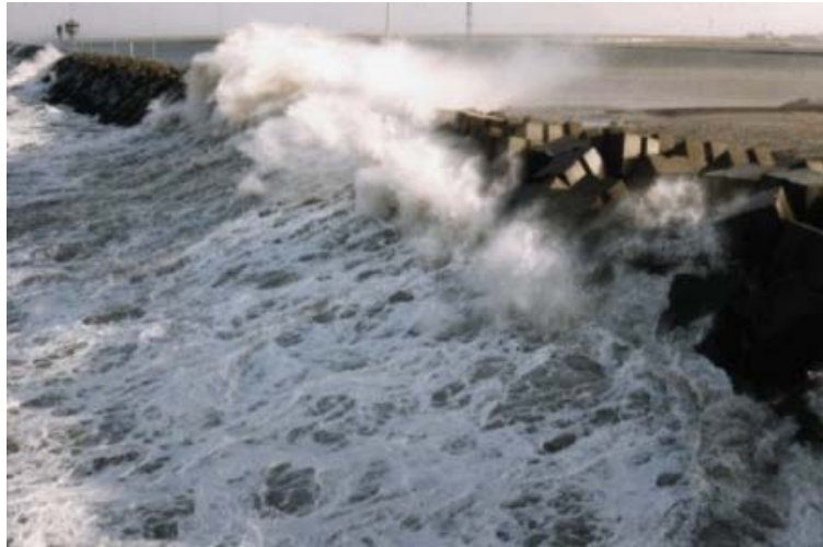
Figure 1.1: Wave run-up and overtopping at Zeebrugge breakwater during (mild) storm conditions (from OPTICREST project, www.rug.ac.be/opticrest ).
