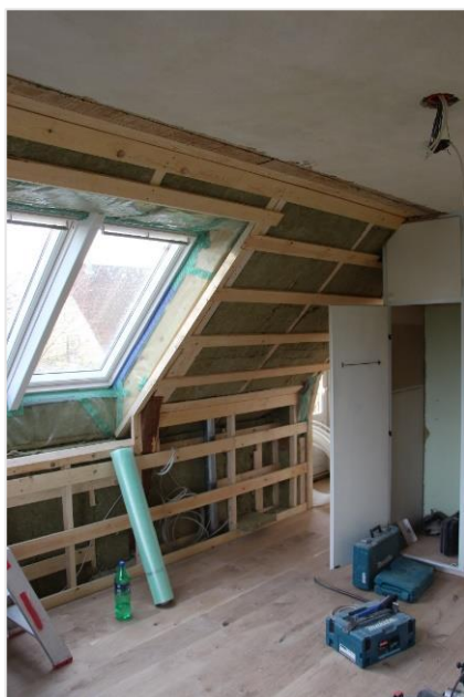
Figure 4-2 Renovation of the external wall and roof of the case study.
