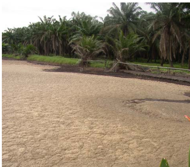
Figure 10.2: Pond for anaerobic treatment of POME (Picture taken in United Plantation Berhad 2006).
