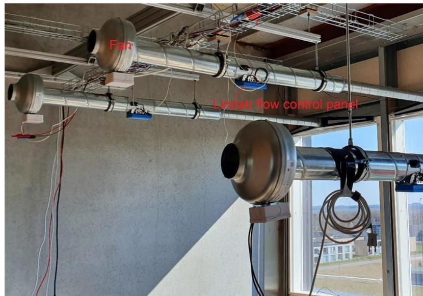
Fig. 6. The exhaust fans for the ventilation system.
