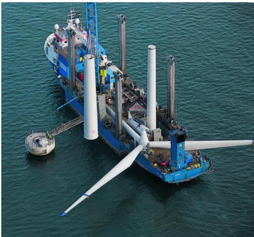
Figure 27: Installation of Roedsand 2 offshore wind farm (2010).
