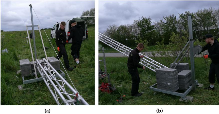
**Fig. L.13:** The portable pole can be raised using a swivel bracket installed in the middle of the base platform. The pole is raised using a steel wire connected to a manual winch system.
