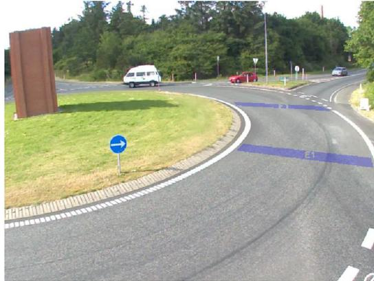
Fig. K.7: Detectors from the vehicle speed study, before the rebuilding.
