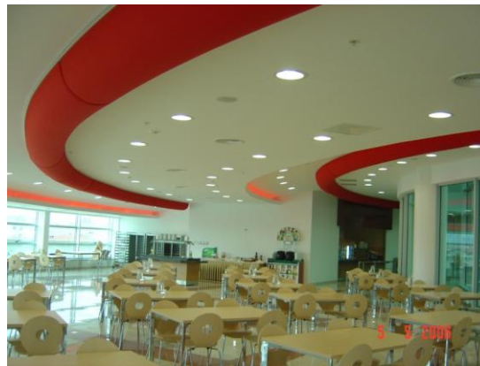
Figure 4. Vertical ventilation from openings in the ceiling. a_o/A \sim medium. The photo shows this type of flow from ceiling mounted textile terminals (KE Fibertec A/S).
