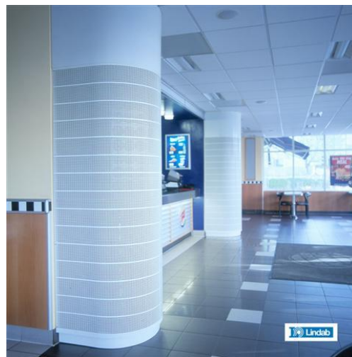
Figure 6. Displacement ventilation. The supply openings are located at a low level, and the return openings are at a high level. The opening supply area is relatively large. The photo shows displacement ventilation diffusers in a restaurant (Lindab A/S).
