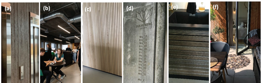
Fig. 6 Photos illustrating some of the details of construction in the Warehouses: (a) wooden-patterned concrete wall in the central hall of each floor in the office unit (b) visible installations on the ceiling in the office unit (c, f) wooden panels on the walls of the offices and
