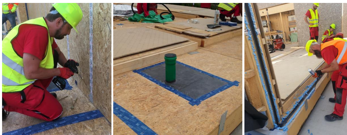
Fig. 3 Air tightness measures carried out precisely by the team members – the construction phase was the first practical experience with structural detail implementation for most of the students.
