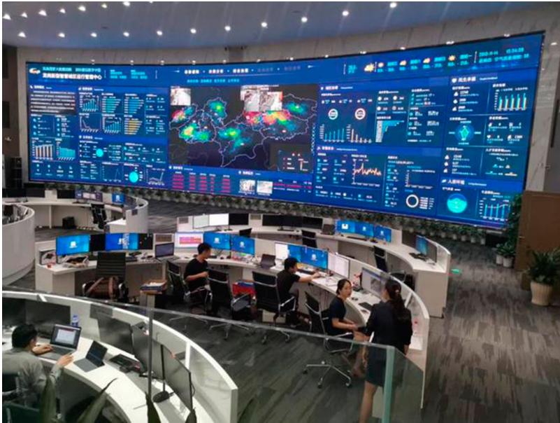
Figure 4. Huawei's Dashboard in Longgang District, Shenzhen. Source: https://www.sohu.com/a/357288371_374240 .
