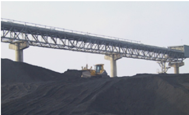
Fig. 7. Coal storage area.
