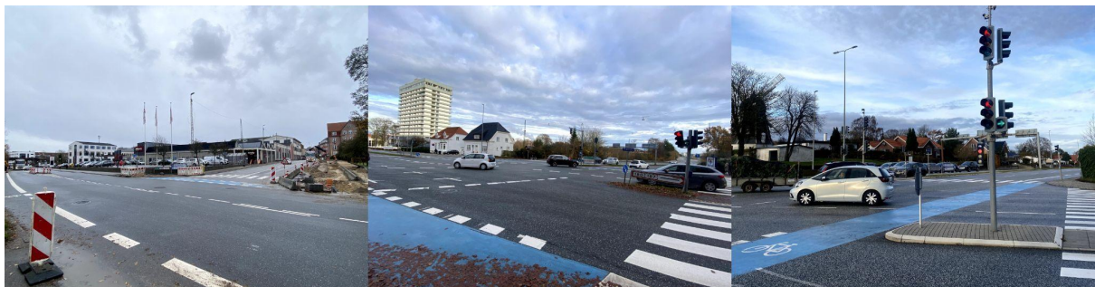
Pictures 37-39: Unfavourable junctions in Aalborg. From left to right: Junction of Peder Skrams Gade and Dannebrogsgade, junction of Vesterbro and Hobrovej, junction of Hobrovej and Over Kæret.
