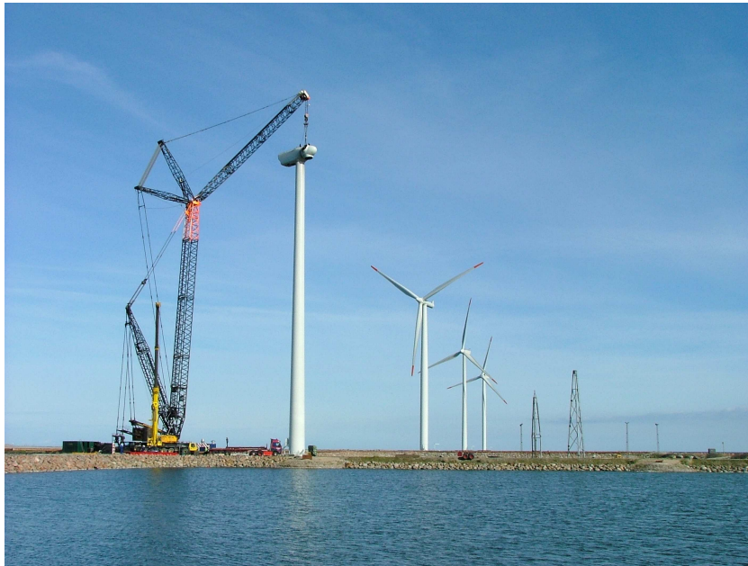
Figure 1.5: Replacement of nacelle in the spring 2005.
