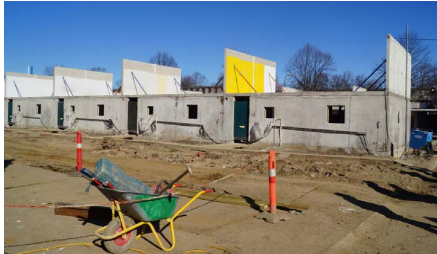
Figure 3. The renovation in Albertslund was comprehensive.
