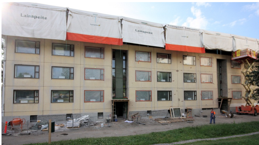
Figure 114. Sahatie 2 during renovation in June 2010. Photo: (Pekka Huovila).
