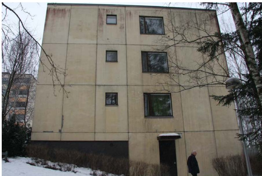
Figure 112. Sahatie 2: four staircases, 42 flats and 3,622 brm 2 in three or four floors. Photo: (Pekka Huovila).
