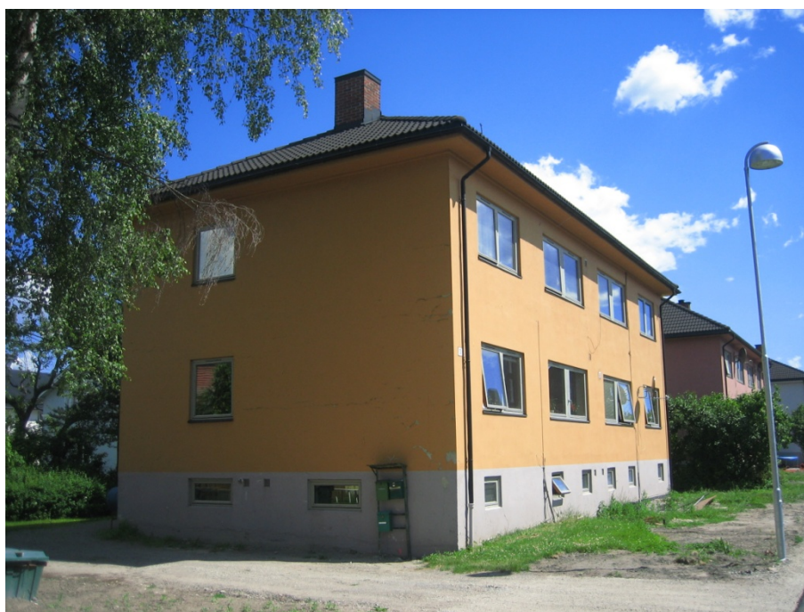
Figure 95. One of the five residential buildings in the case study. Photo: (Anders-Johan Almås).
