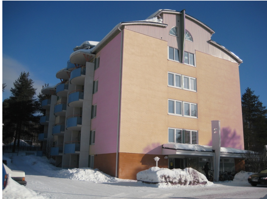
Figure 119. The neighbouring building DAS II after refurbishment. Photo: (Jyri Nieminen).
