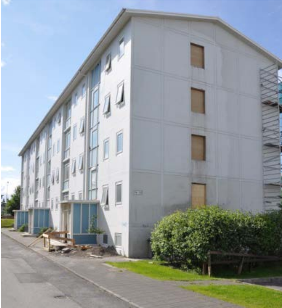
Figure 108. North view. New window openings have been cut out on the gable wall (during refurbishment). Photo: (Björn Marteinsson).
