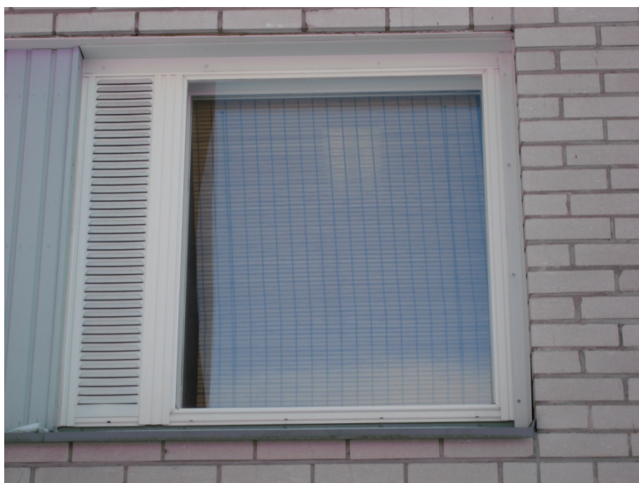
Figure 122. The windows were upgraded in 1995. Photo: (Jyri Nieminen).
