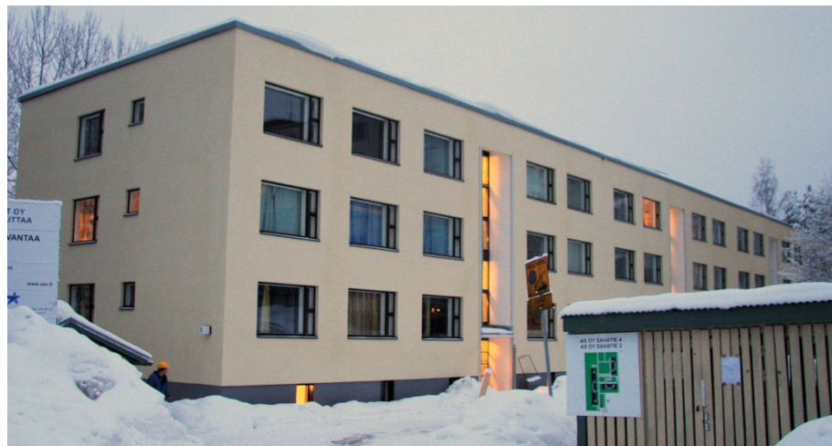
Figure 116. Sahatie 2 after refurbishment in January 2011. Photo: (Pekka Huovila).
