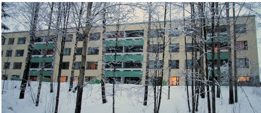
Figure 117. Sahatie 2 after refurbishment in January 2011. Photo: (Pekka Huovila).
