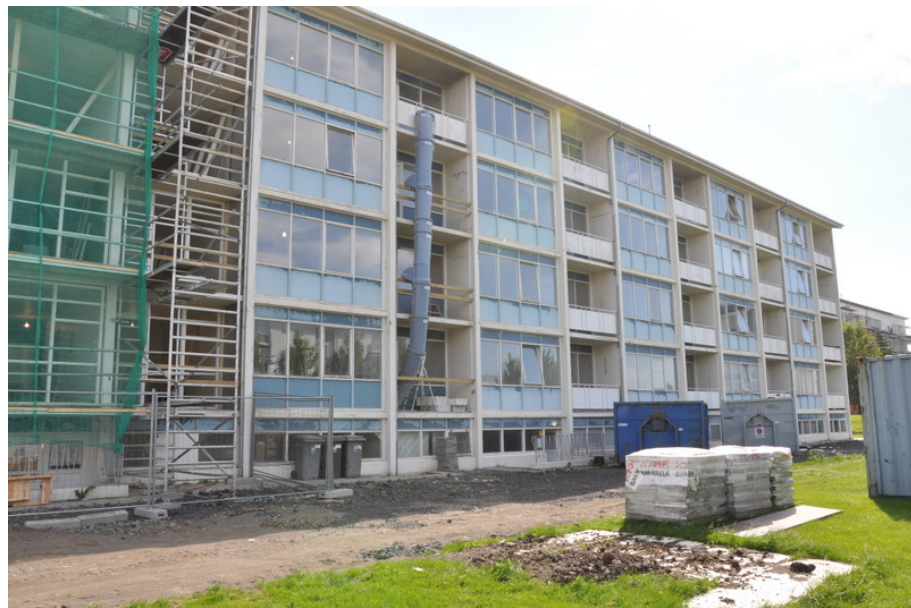
Figure 107. Meistaravellir 19-23. South view (during refurbishment). Photo: (Björn Marteinnsson).
