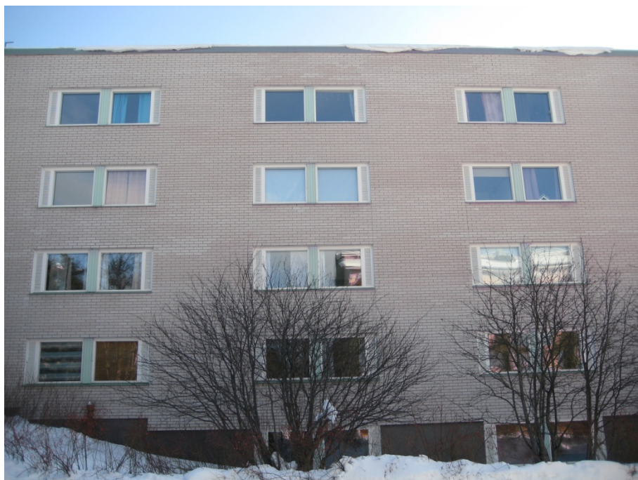
Figure 121. DAS III has a ventilated masonry facade. Photo: (Jyri Nieminen).
