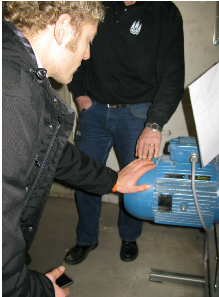
Figure 76. Circulation pumps are replaced mostly by low-energy models, which also facilitate and interface to the intranet. Photo: (Peter Vogelius).
