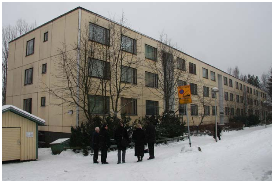
Figure 111. Sahatie 2 Vantaa in February 2009 before the refurbishment started. Photo: (Pekka Huovila).
