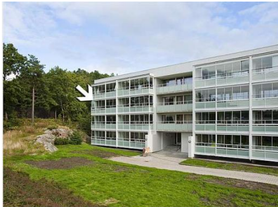
Figure 105. West façade of the case building after refurbishment. Photo: (Kruse Smith).
