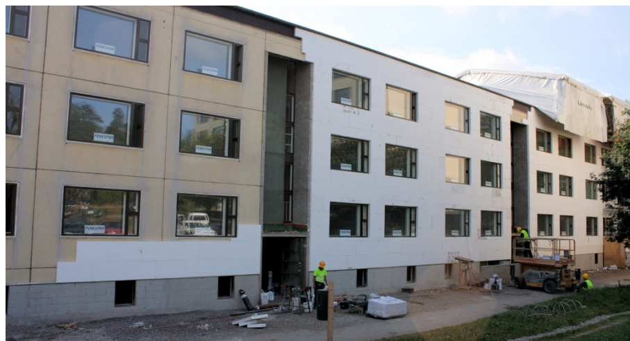
Figure 115. Sahatie 2 during renovation in August 2010. Photo: (Pekka Huovila).
