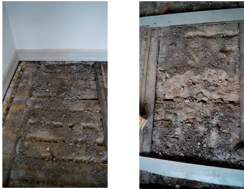
Figure 17 condition of wooden flooring during the renovation
