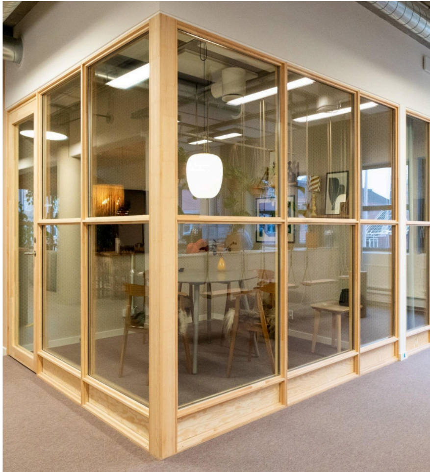
Figure 14 - Indoor wall panels made from repurposed IGUs (A:gain, n.d.)
