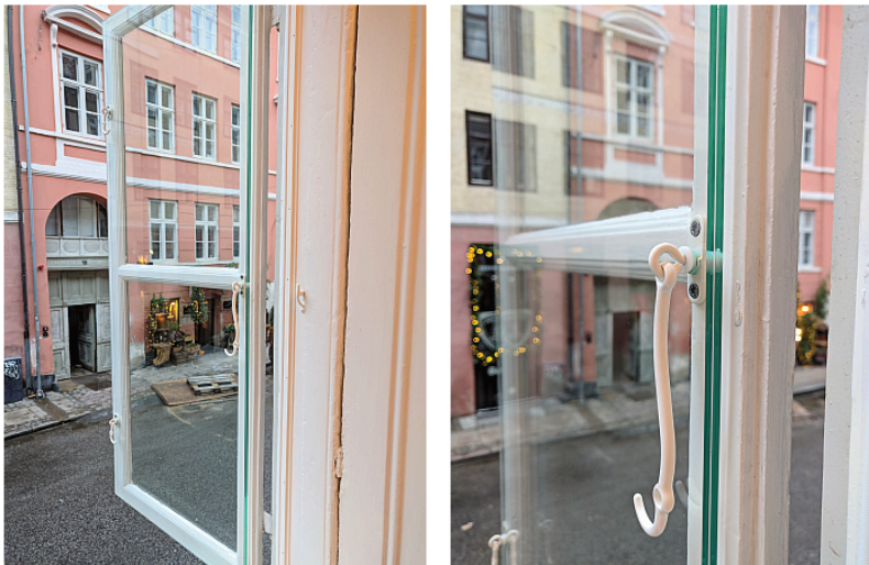
Figure 15 - Windows refurbished with a secondary glazing (Optoglas, n.d.-b)
