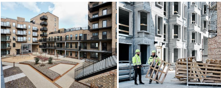
Figure 4: Pictures of the building (left) and wood sorting at the ‘Waterside Buildings’ project (right)
