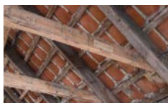
Roof tiles Aggregate
