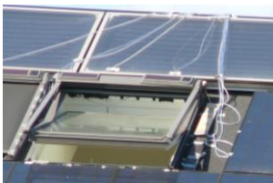
Figure 4. Pressure taps location on site (17.1° open)
