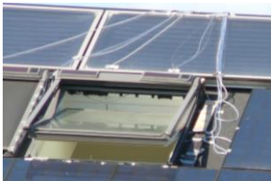
Figure 4. Pressure taps location on site ( 17.1^\circ open)
