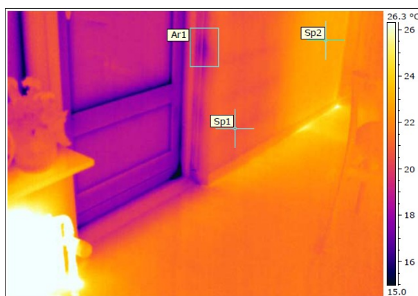
Figure 5. The transition between the wall and the floor is acceptable.
