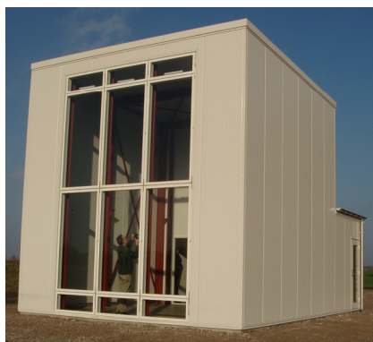
Figure 1. South (DSF) façade of the test facility.
