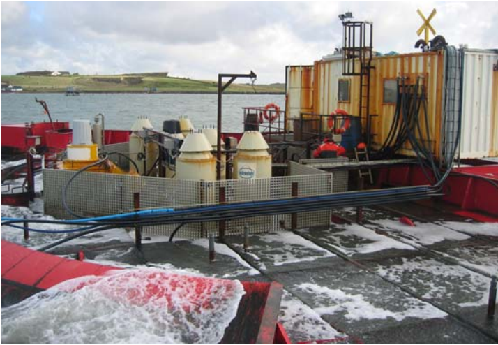
Figure 5. Trash rack with 5 x 5 cm openings enclosing the turbine area.
