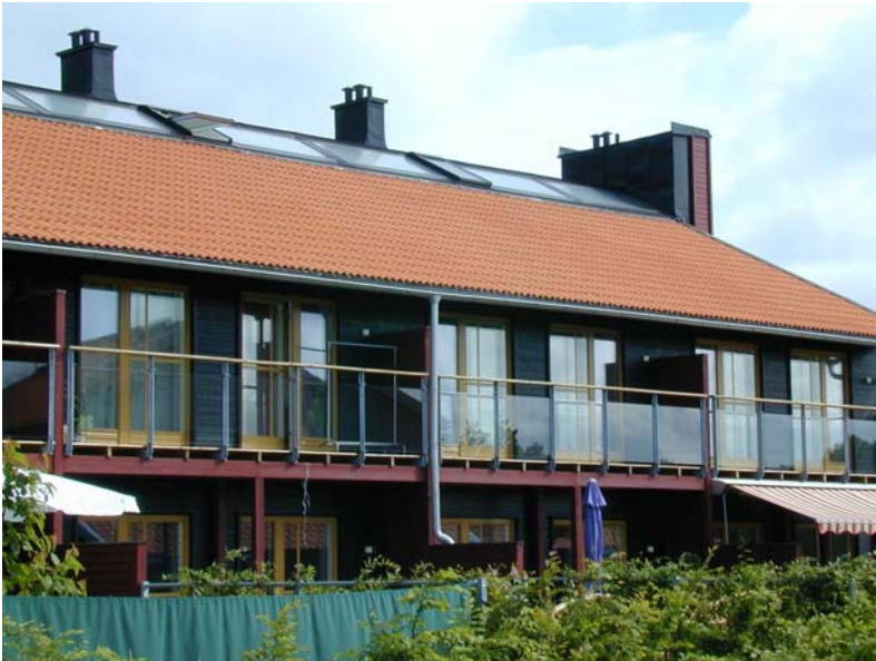
Figure 1. Passive houses at Lindås Park with solar collectors at the roof. Photo: Inger Andresen.
