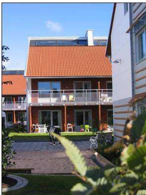
Figure 3. Passive houses at Värnamo with solar collectors at the roof. Photo: Ulla Janson.
