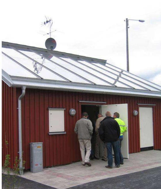
Figure 4: Solar panels in Frillesås
