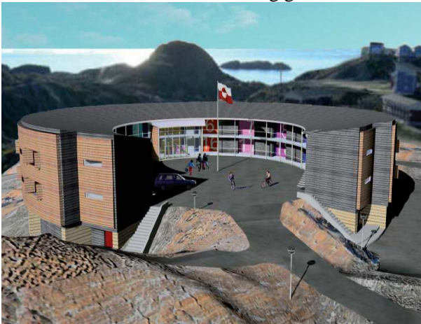
FIG 1: Dormitory building in Sisimiut, Greenland
