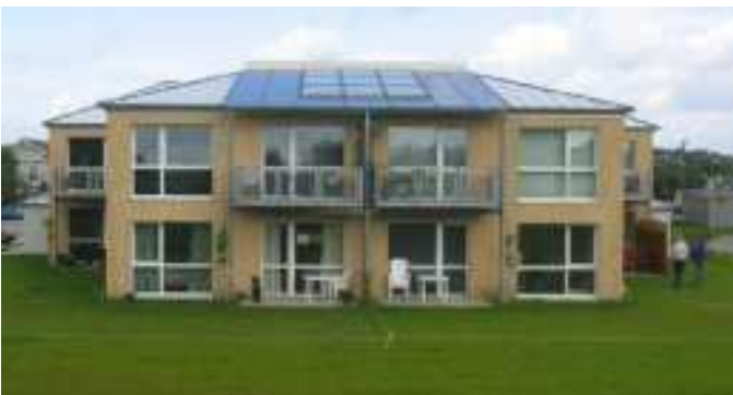
Figure 5. South facing facade of the Rønnebækhave house. Photo: Cenergia.
