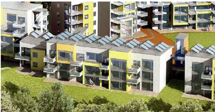
Figure 10. Left: The Løvåshagen passive houses with south facing solar collectors on the roof, illustration: ABO Architects. Right: System layout, Illustration: Skjøelberg.
