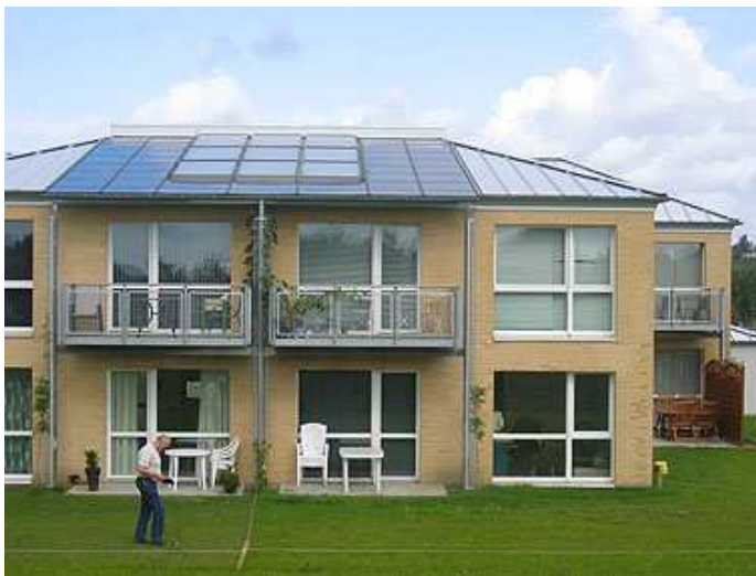
Fig. 1.1. 50 m 2 PV-modules in Rønnebækhave II is mounted in the roof facing south in connection to a solar collector area of 28 m 2 .
