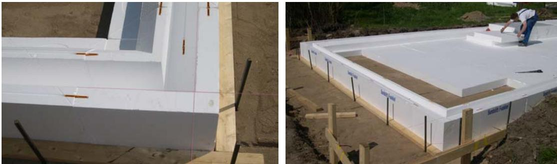
*FIG. 3 a): left, prefabricated EPS elements mounted as the strip foundation and held together with large staple-shaped pieces of plastic, b): right, 300 mm EPS, mounted as two layers on top of the base of stamped gravel bordered by the strip foundation, serving as the insulation layer beneath the concrete slab.*
