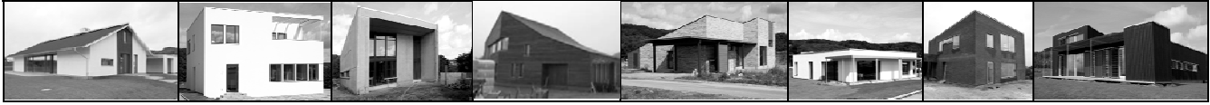
Figure 1: Overview of the Comfort Houses that fulfils the German passive house standard [1].
