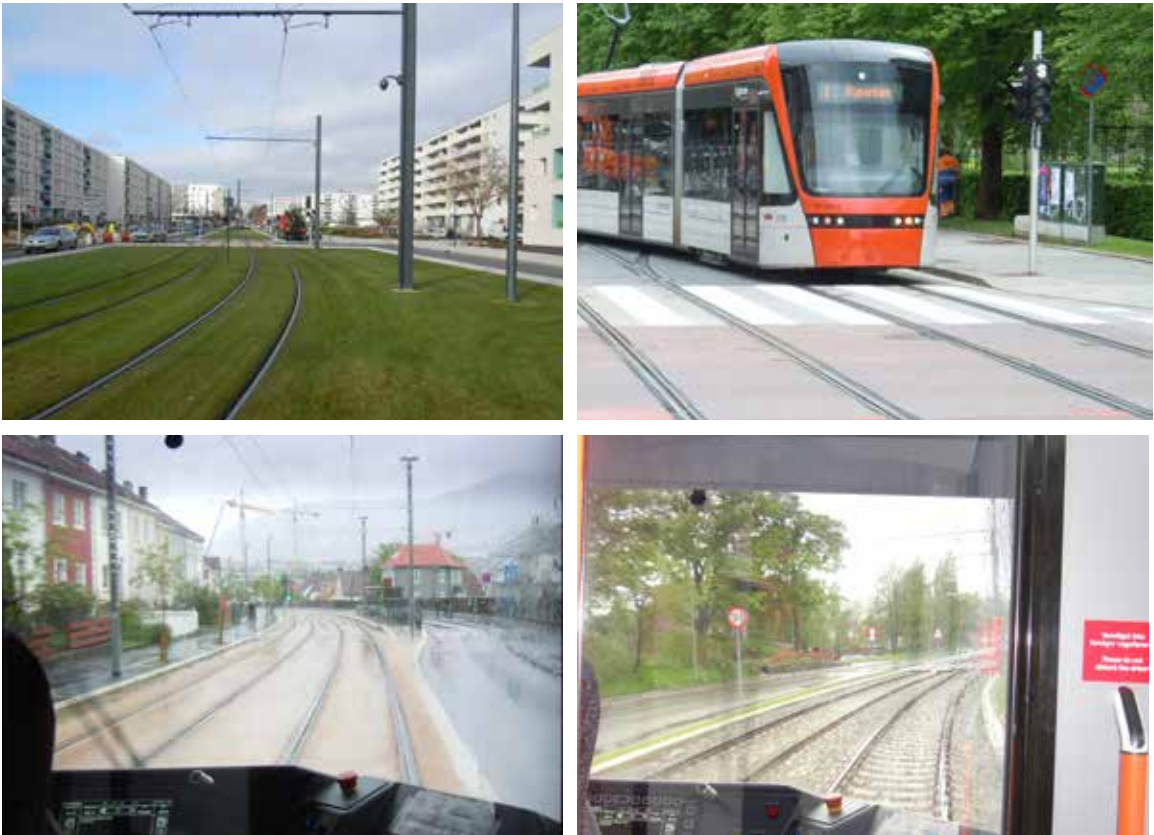
Figure 8: Different identities of the light railscape provided by a change in pavement. Above left: green tracks on 70% of the line in Angers, and on selected areas in Bergen. Above right: red pavement on the urban parts in Bergen. Below left: Yellow tracks in segregated tracks along existing infrastructure. Below right: Heavy rail tracks on the part completely segregated from the city. In this sense the materiality of the tracks and the pavement provides and mediates different identities in different districts along the line. (Photos by author).
