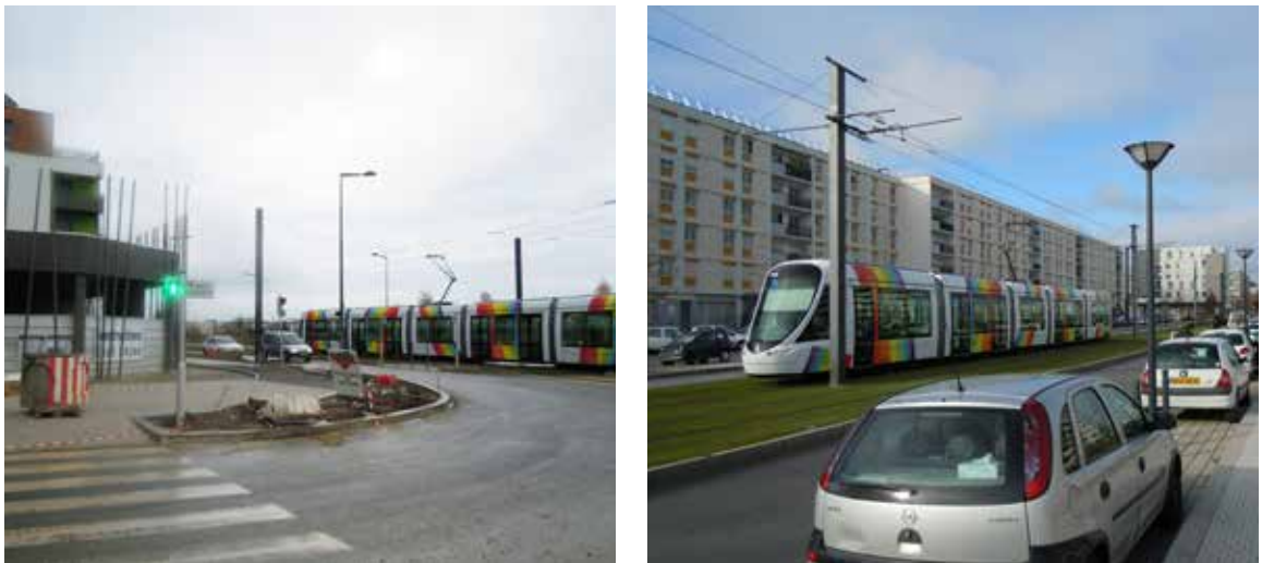
Figure 5: Two diverse urban areas connected by the light rail in Angers. Construction of the new district around Plateau Mayenne (left) and the socially and physically deprived housing area in La Roseraie (right) has provided a physical upgrade and a new link between these two diverse districts by securing an equal aesthetic and physical upgrade or redesign (Photos by Author).
