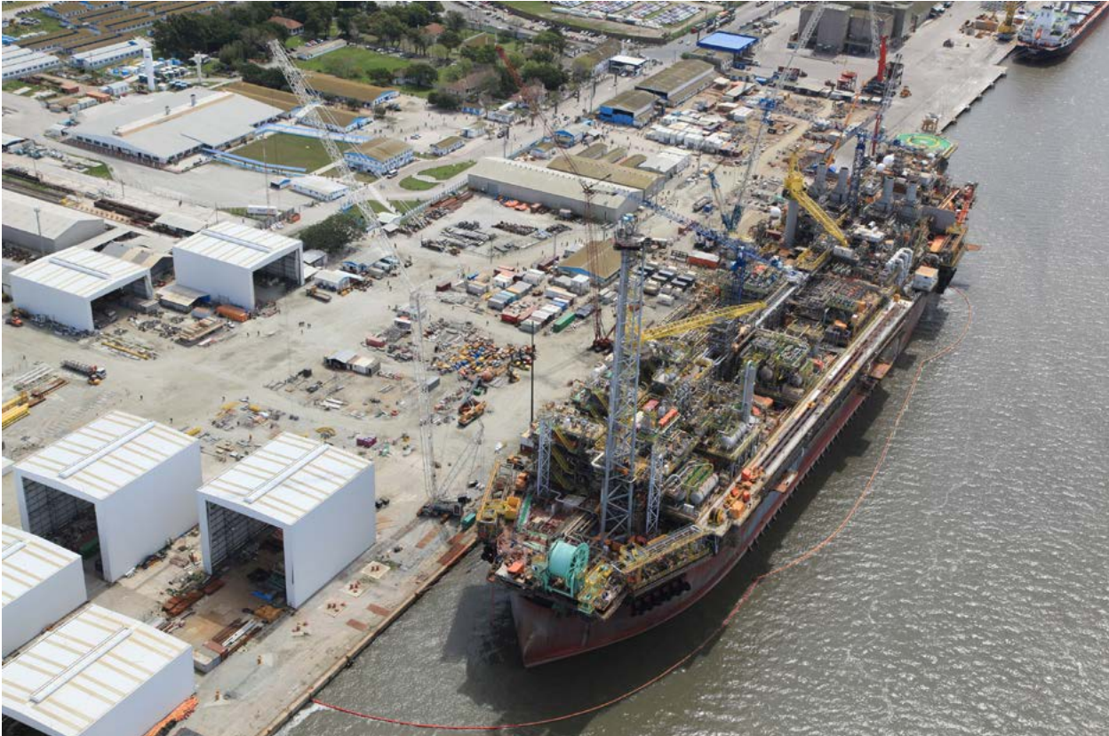
The supply chain of multinational energy corporation Petrobras has been a focus of public procurement of innovation policy in Brazil. Photo: Petrobras
