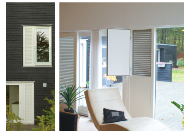
Fig. 39. In this house, shutters are included in the window design. The windows cannot be opened; instead ventilation takes place by using a hatch behind the shutters. The shutters can be opened or locked as required.
