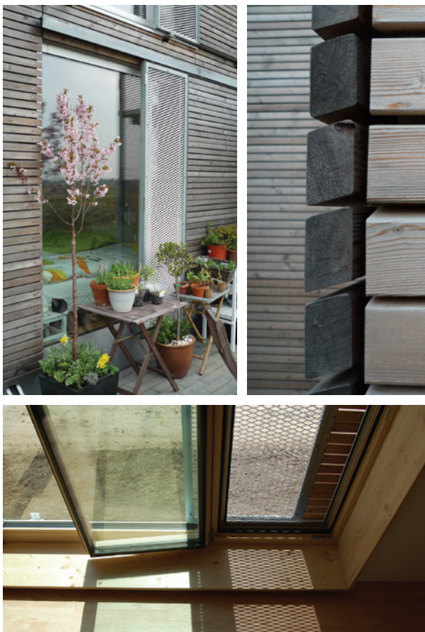
Fig. 25. Solar shading is an important element in ZEB design. For the terraced houses Lærkehaven in Lystrup, Denmark (2008, Architect Herzog + partner) manual shutters on southern, eastern and western facades facilitate a balanced utilisation of passive solar heat. Other strategies applied in the project are highly insulating and airtight building envelope, heat accumulating ceiling panels with phase change materials, use of LED lighting and use of FSC certified wood (Boligforeningen Ringgården 2014).
