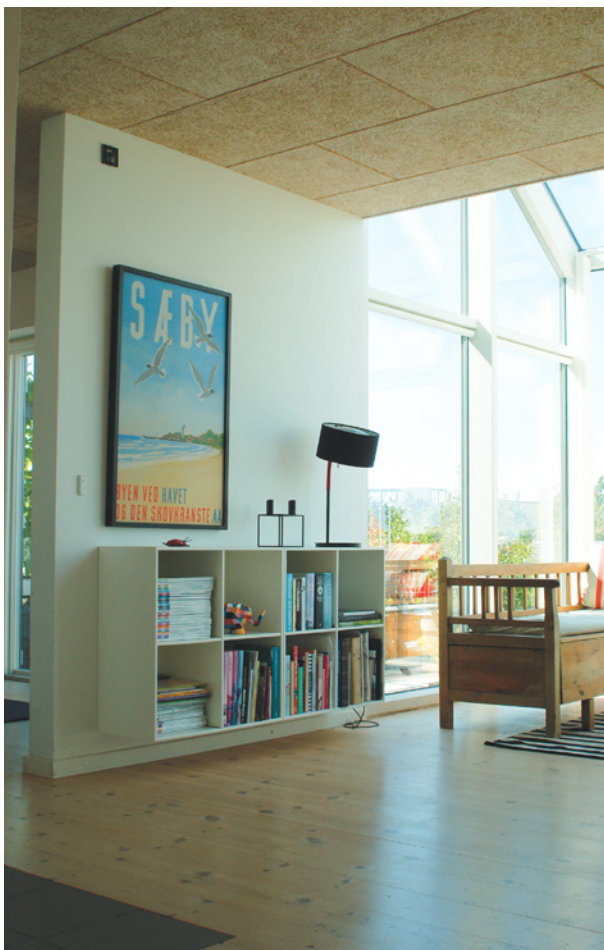
Fig. 44. Today, many houses are built with large open spaces and hard materials (e.g. tiled floors, smoothly plastered walls and ceilings), which often results in poor room acoustics. Sound absorbing acoustic panels (as in the picture) is one way of achieving better room acoustics. Carpets, soft furniture and pictures may also help.
