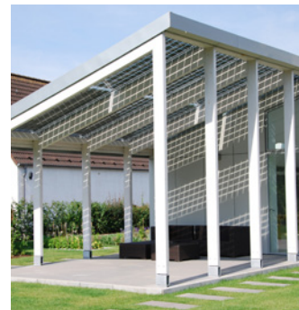
Fig. 64. Solar PV used for glass covering of outdoor space. Light active house, Germany.
