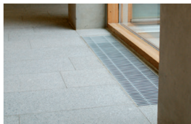
Fig. 40. Floor convector.
