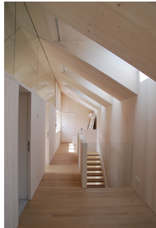
Fig. 31. In Sunlight House, Austria, transverse lighting is ensured by a glass construction in the upper part of the partition. This also adds to the spatiality of the corridor.
