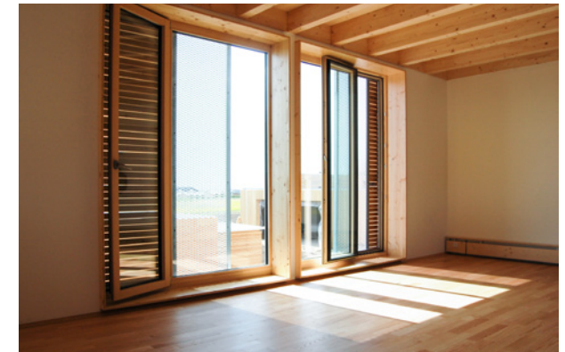
Fig. 36. Solar shading is essential for the spatial experience. In this house in Lystrup, Denmark, exterior lamellas and perforated steel plates in combination control the supply of passive solar heat.
