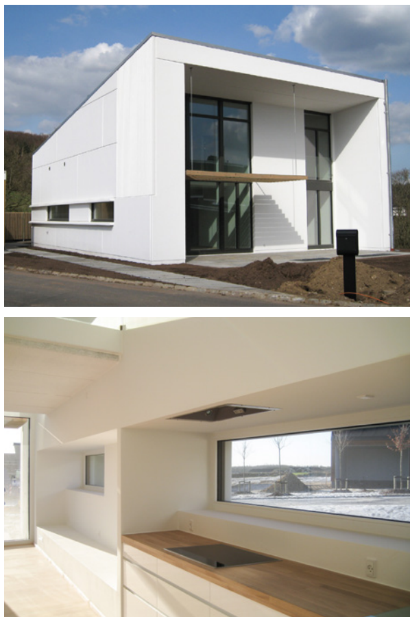
Fig. 26. The comfort house at 45 Stenagervænget, Vejle, Denmark (Hundsbæk & Henriksen Ltd and Ravn Architecture), which was built as a passive house, has a glass-covered atrium as its focal point. The atrium is a source of daylight and by means of highly placed windows in the atrium and split-level floors, natural ventilation may be increased on hot days. Rooms lit from both sides, soundproof floor structure with acoustical surfaces and low-energy appliances are other applied strategies.
