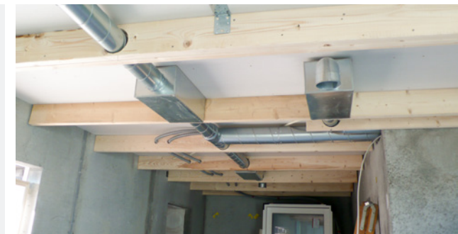
Fig. 37. Battens attached below the load bearing floor structure may ensure space for ducts and silencers. Sheathing is mounted underneath.
