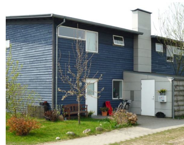
Fig. 38. A solar chimney may increase natural ventilation by thermal buoyancy.
