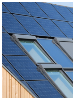
Fig. 63. Solar PV panels used as roof surface. Sunlight House, Austria.
