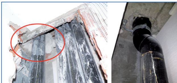
Figure 10.9. Waste water pipes embedded in mortar (left). Changes of direction in waste water pipes (right).
