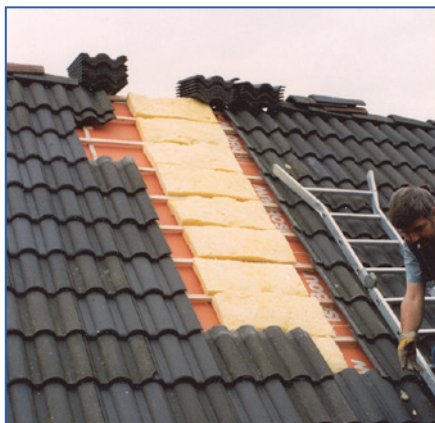
Figure 10.29. No mineral wool sound barrier above partition wall in combination with roof elements with rigid thermal insulation (PUR, PIR, EPS) leads to a decrease of 5 – 10 dB in airborne sound insulation between rooms.
