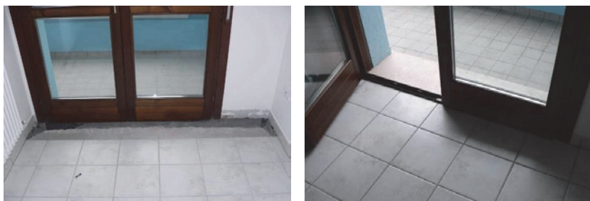
Figure 10.5. View of the French window area with the first row of tiles and floating mortar removed (on the left) and after the repair (on the right).
