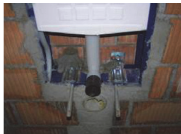
Bad workmanship Rigid contact (mortar) between sanitary equipment and wall
