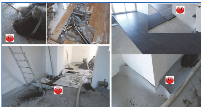
Figure 2.36. Bad execution of a mounting floor; sharp objects can puncture the elastic interlayer. Foils should have sufficient overlap and should be taped together. The against the wall upwards turned elastic interlayer should only be cut off after the tiling (if before, the tiles or the glue can make a hard connection with the wall, seriously diminishing the impact and airborne sound insulation of the floating floor).
