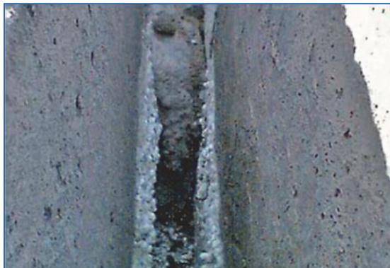
Figure 26.14. Casting waste between separated floor plates for row houses causing sound bridges.
