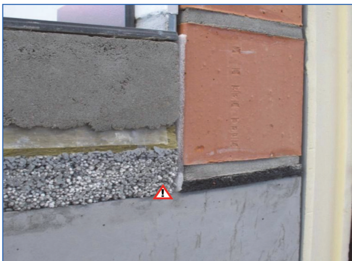
Figure 2.12. Detail of concrete slab with floating floor and acoustic strip (Sonic strip, Wienerberger – CDM). It is important to put a border resilient strip before executing the levelling screed to avoid a hard contact between the concrete slab and the brick wall!
