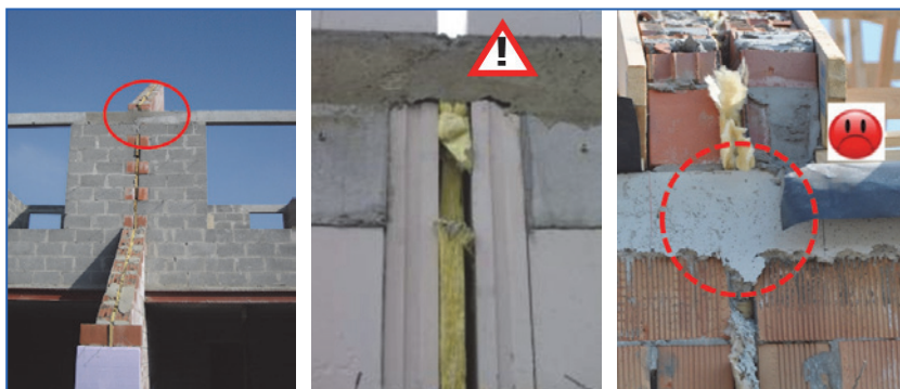
Figure 2.7. Hard connections (continuous floors, concrete beams but even small metal ties can largely reduce the sound insulation; the party wall loses its acoustic double wall behaviour and extra flanking transmission will occur.
