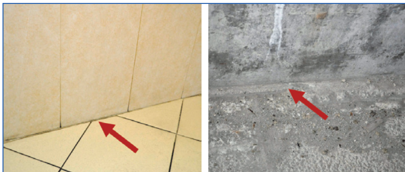
Figure 22.8. Two examples of workmanship errors on floating floor: rigid contact between ceramic tiles on floor and wall (left), gap around a floating floor intentionally filled with mortar (right).
