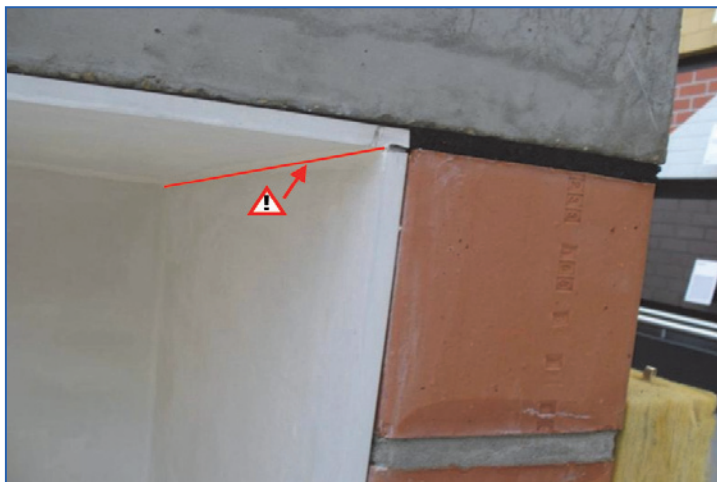
Figure 2.13. Detail of the acoustic strip below the concrete slab and on top of the wall. It is always important to cut the plaster at the junction between the brick wall and the concrete slab to avoid cracks (different thermal dilatation), but when using acoustic strips, it should be cut completely down to the acoustic strip and filled up with silicones to avoid a “vibration bridge”.
