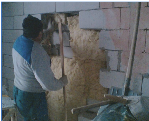
Figure 11.7. Stuffing the cavity with glass wool – a typical workmanship error of constructing double walls and furrings.
