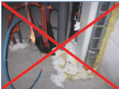
Figure 8.12. Example of problems related to piping system going through separating floor slab.
