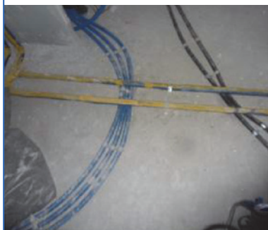
Bad workmanship Pipes crossing each other
