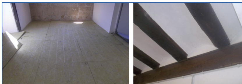
Figure 25.26. Left. Image of the construction of the floating floor. Note that the flanking strips are missing in this image. Right, view of the bottom face of the floor after the retrofitting.
