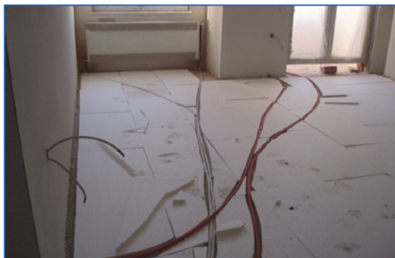
Figure 15.7. Typical error in workmanship – broken insulation.
