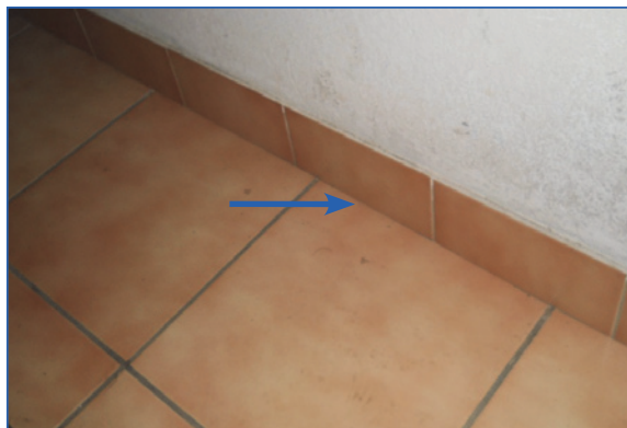
Figure 24.10. An example of a rigid contact of wall and screed via floor ceramics.
