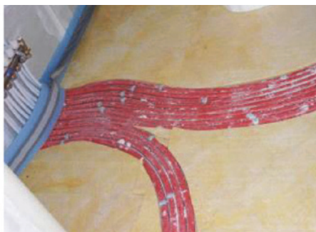
Bad workmanship Tubes in resilient layer
