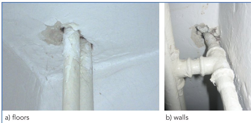
Figure 21.21. Typical errors for cross pipes.
