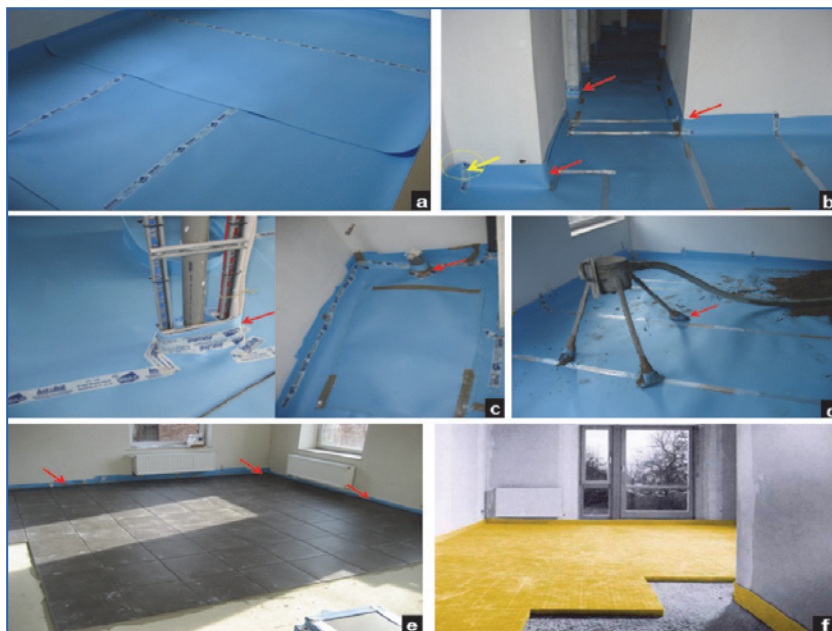
Figure 2.35. Correct mounting of a floating floor.
