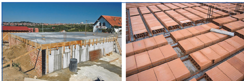
Figure 3.8. The most common floor slab designs: reinforced concrete (left) and brick system (right).
