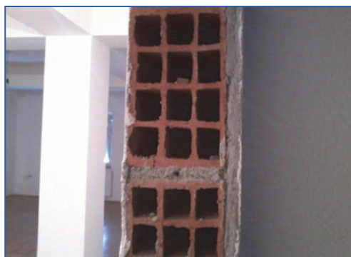
Figure 15.11. Typical errors in workmanship – irregular mortar layers.
