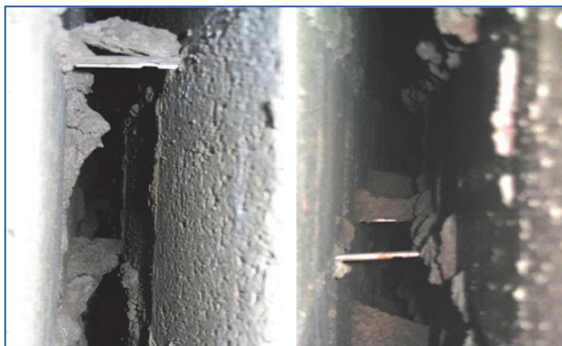
Figure 29.6. Example of poor workmanship in cavity separating walls, showing incorrect wall ties and also mortar being allowed to collect on ties (these provide strong acoustic bridges which weaken the sound insulation performance by 6 dB to 10 dB).
