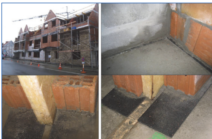
Figure 2.14. Application of acoustic strips below brick walls (party wall below) and concrete blocks (the elevator shaft). The acoustic strips (CDM, Sonic strips) have only a limited deformation (2 mm under the weight of the building, almost no creep in time).
