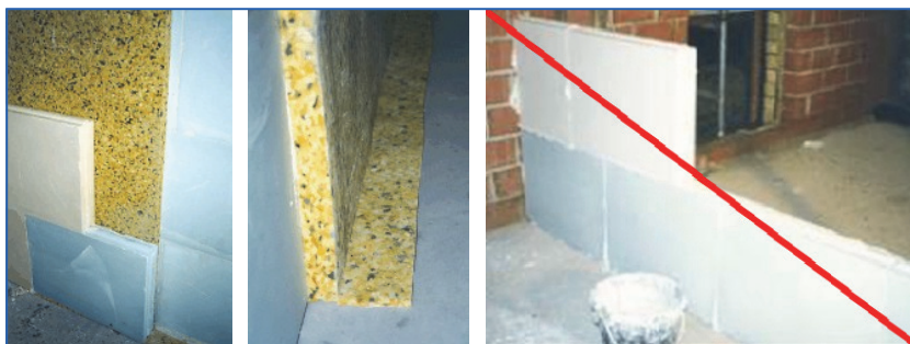
Figure 2.21. Gypsum block walls need to well disconnected from the surrounding structure.
