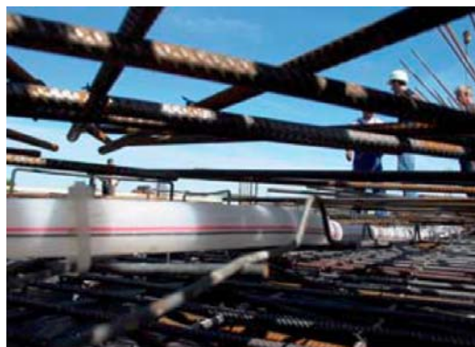
Figure 4: Close-up on the pipes during the construction phase (Source: BINE Themeninfo I [2007])
