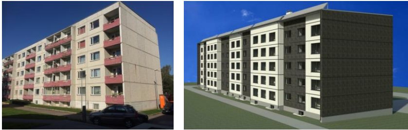
Fig. 1 Photo of the pilot building (left) and the designed solution after the renovation (right) [16].
