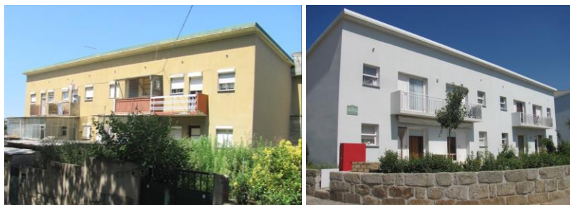
Figure 1. General aspect of the building before and after the renovation
