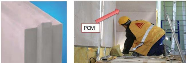
Fig. 3 Rigips Alba Balance plasterboard used in EFdeN house (source: rigips\_alba\_balance\_infobro\_de\_low\_en\_korr\_arial.pdf)
