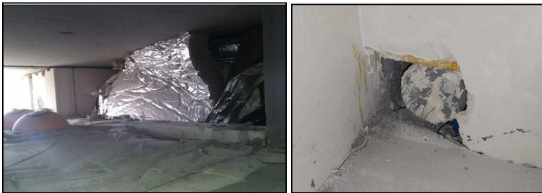
Fig. 5 Chimneys top with gaps between chimney walls and ventilation duct (building #1, left) and large openings between dwellings and shafts (building #2, right)
