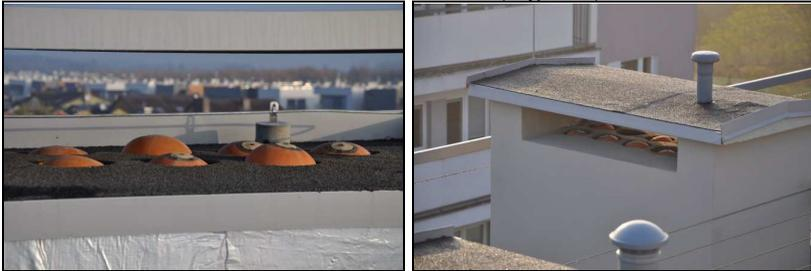
Fig. 4 Extract ducts closed with use of inflatable inner rubber bladder, building #1
