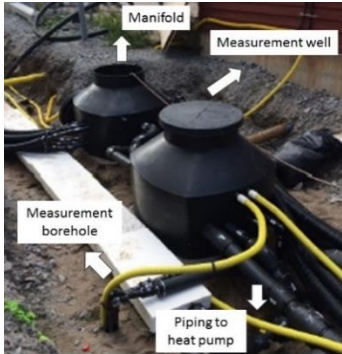
Figure 7-a Manifold and measurement well
