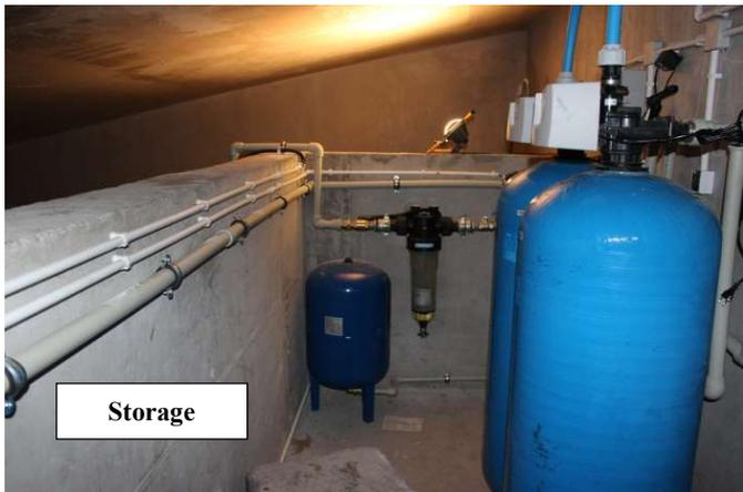
Fig.3 Rainwater harvesting system (storage, filters) in the multi-dwelling Urban Building in Warsaw/Poland (photo by M. Lipska)
