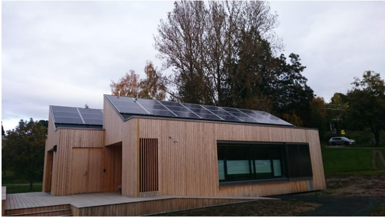
Fig. 1. The Living Lab in Trondheim viewed from the South. Solar collectors are integrated in the south-exposed façade, right next to the window.
