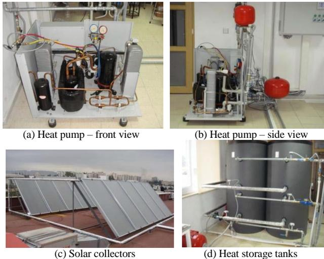
Fig. 1 Components of solar assisted water source heat pump system
