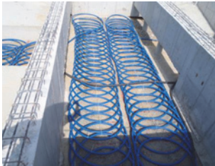
(1) Rolled pipes are set as they are
