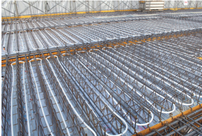
Fig. 2 The piping laid in the concrete slab
