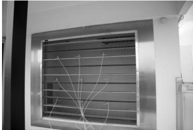
Fig. 7 Multipoint tracer injection upstream on the roof level of building 2
