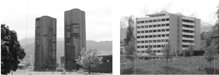
Fig. 1 Building 1, at left (Allmend Hoch2, Lucerne) and building 2 (staff accomodation building of Lucerne Hospital)
