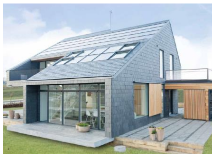
Fig. 1 South East view of the building
