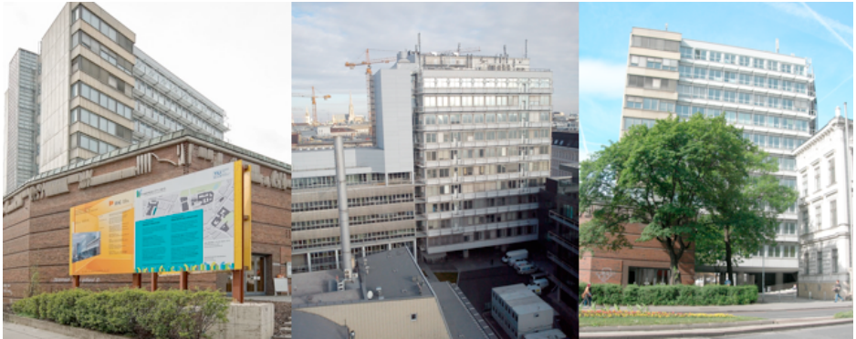
Fig. 1 - Plus-plus-energy office building before the refurbishment [1]
