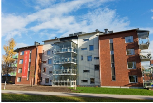
Fig. 1 Photograph of building A
